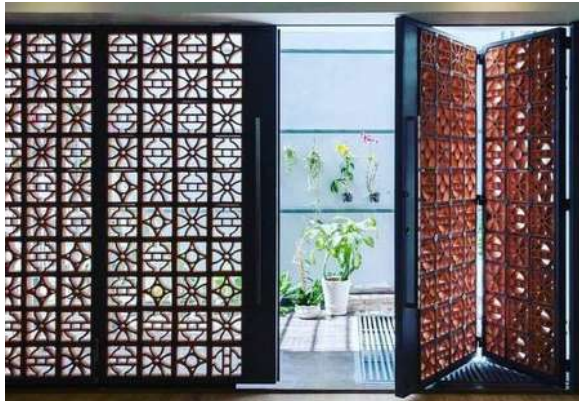
Pivoted Terracotta jali wall as a Semi-transparent separation between lift lobby and shared space
