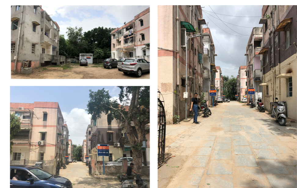
PICTURES OF THE SITE, CURRENTLY THERE ARE 4 BLOCKS & 42 HOUSES IN TOTAL
