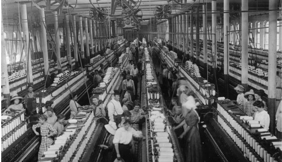
Prefabrication in factories
